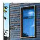
(M2) Aluminium framed cladding
